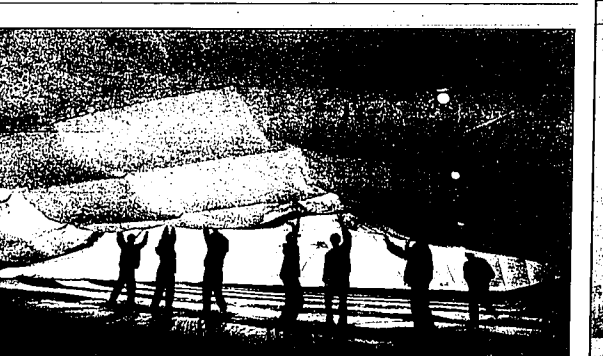
Volunteers hold up the covering on the Twin Falls Municipal Pool as the large bubble roof is inflated on Saturday.
