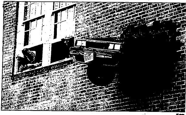
Students at Central School in Libby, Mont., look out a second story window next to a car's front and mounted on the wall Wednesday as part of an art project.
