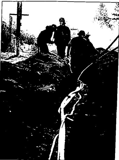
Bret Gilbreth leads a crew from Dayley Construction in running fiber optic cable lines through Burley on Parke Avenue.
