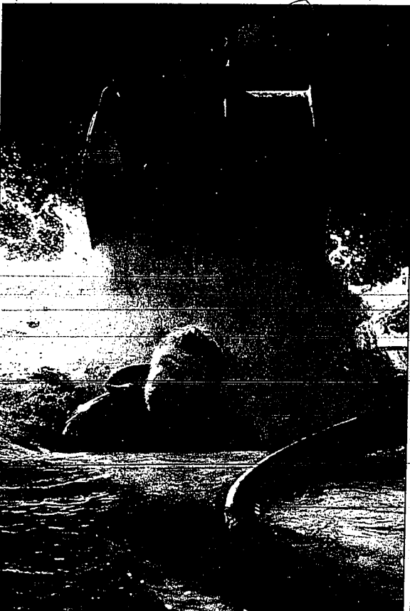
Wally Hendrick struggles to fit a repair clamp on a broken water main in the 200 block of Eighth Avenue North Wednesday afternoon. The pressure on the pipe was so severe crews used a backhoe to prevent water from spraying over the roof of a two-story house.
