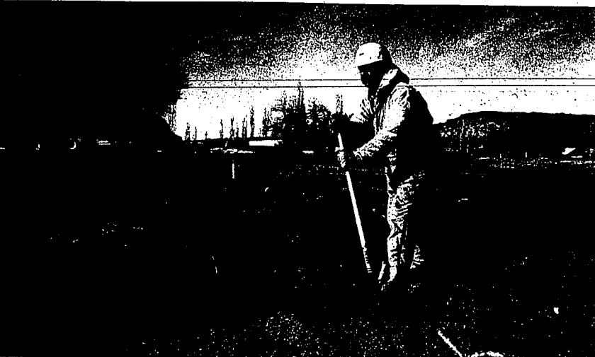
Jerry Santillanes, worker for H-K Contractors Inc., oversees the digging of the old pipeline that runs through Canyon Springs Golf Course.
