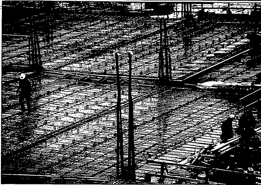
Work continues Tuesday on a new parking garage on the Boise State University campus.
