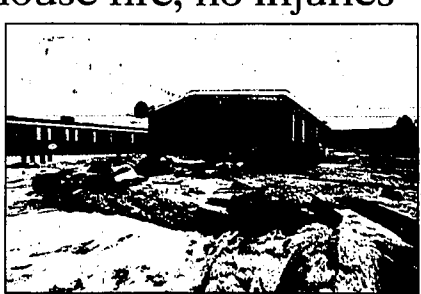
Investigators suspect arson in a Monday fire that caused an estimated $50,000 damage to a Burley home.
