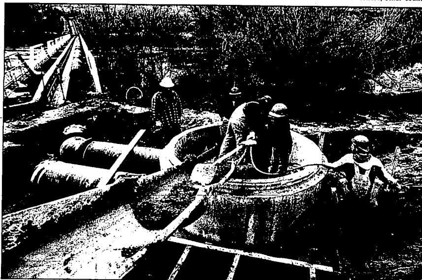
A construction crew pours concrete over a new water pipe near the Snake River on Monday. When the project is finished, more than 2,000 feet of pipe will be replaced from the springs that are the city's main water supply to a pumping station in the canyon.
