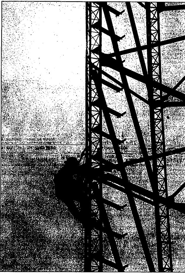
A worker for Christiansen Griffith General Contractor bolts together a section of a tower on Canyon Street in Twin Falls on Monday. The tower is for the Nextel company and will be used for digital cellular phone communications. When complete, the tower will be about 300 feet tall.
