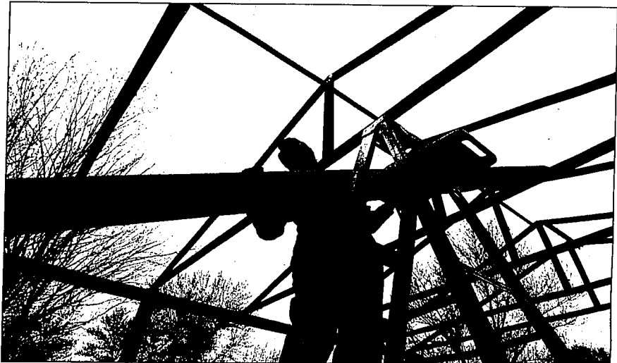
Todd Anderson of the Twin Falls Parks and Recreation Department works on a shelter in Mammoth Park on Tuesday afternoon. The shelters should be completed within the next two weeks.
