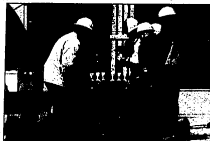
Electrical workers work Wednesday morning at Bonneville Power Administration's Riverton substation. The workers were trying to restore power after a backup line failed at around 6 a.m. Power was restored to most areas by 11:15 a.m., but some parts didn't receive electricity until 2:30 p.m.
