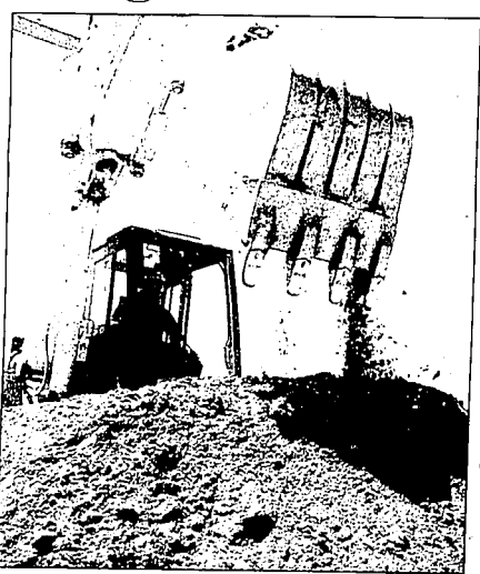
Brian Kinney operates a backhoe for some work the city of Rupert is doing in preparation for road improvement projects.
