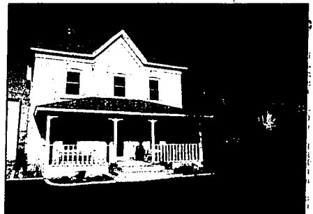
Sally McMurray talks about the home she and her husband recently remodeled. McMurray's home is a new addition to today's historic home tour in Oakley.
