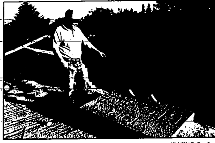
Jim Muhlstein points to one of the title stones taken from the old Oakley Grade School. Demolition of the building is now under way with the roof and third floor already gone.
