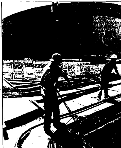
Telephone workers pull some of the thousands of miles of phone cable Sunday that is being used for the Democratic National Convention in Los Angeles.
