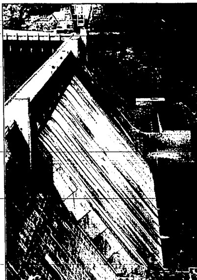
Cars driving on top of the spillway of the Grand Coulee Dam in Washington are barely visible in this May photo. It's 550 feet high, 500 feet wide at the base and 30 feet thick at the two-lane road on the crest.
