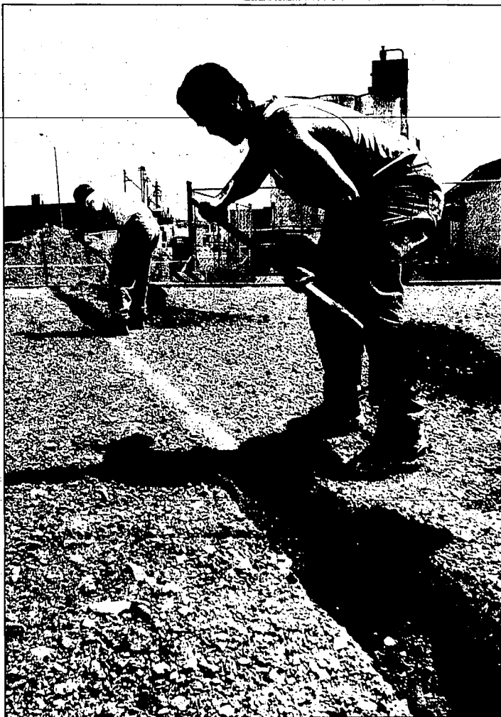
Travis Klundt and Dusty Jenkins work for Shane's Plumbing on the construction of the new Treasure Cove, a family entertainment center in Old Towne Twin Falls.
