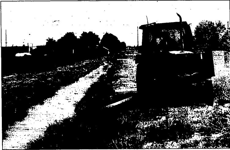
Glenn Boyles, a maintenance worker for Twin Falls Canal Co., uses a tractor with a mower to trim the edges of canal banks.
