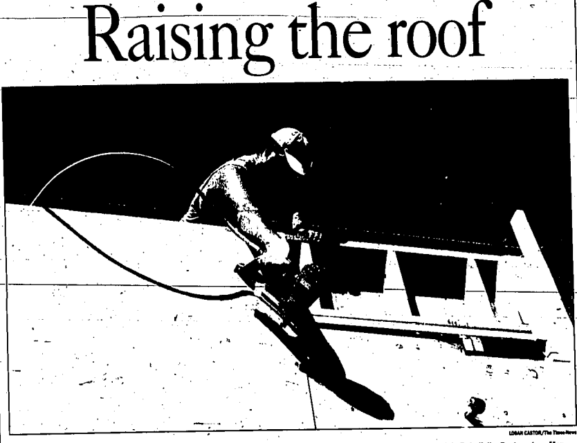
Wes Smith, of Darren Hall Construction, works on the roof of the former Gendeppe restaurant on Blue Lakes Boulevard North in Twin Falls. Restaurateur Max Humphries of Maxie's Pizza and Pasta is turning the building into an Italian restaurant.
