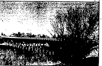
A new weight limit will be in place for Jackson Bridge Monday. Weakening supports in the substructure worried local authorities, and the bridge's weight limit will be lowered from eight tons to five tons, and semi trucks and buses will be banned. Rupert. Last year, the bridge received a rating of 49.9, on a scale from one to 100. Tests done Please see BRIDGE, Page A6
