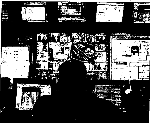
Greg Savage, a network operations analyst for Zama Networks, monitors every aspect of Zama's building and operations, including its own in-house Internet server farm, in the Network Operations Center in Tukwila, Wash., recently. More than two dozen 'server farms' - data centers that store the content and switch the traffic of the Internet - are planned for the Seattle area.
