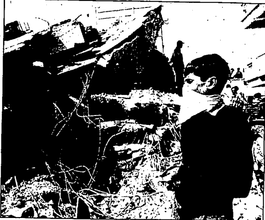
A volunteer wears a face mask while passing by the rubble of a school which collapsed in Ahmedabad, Saturday. Police said 15 children were still trapped inside the rubble from which they had removed 16 bodies and rescued six surviving children.
