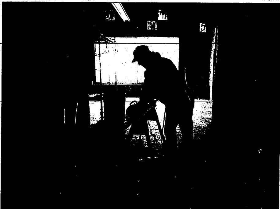
Rick Skeen cuts a piece of lumber in the new inside-sales office at The Times-News' annex building on Main Avenue in Twin Falls. Among other things, the remodeling project will put a historic-style customer door and redesigned windows on the Main Avenue frontage and add a tiled reception area and a bathroom.
