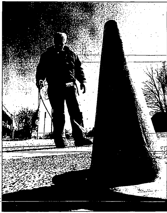
Loran Gillespie uses a torch to melt a section of hot tape on a crosswalk outside of Bickel Elementary School in Twin Falls Wednesday. With all of the schools in town, there are about 250 school intersections and each one must be re-striped every four years. The street department uses the plastic tape rather than paint because it lasts longer.
