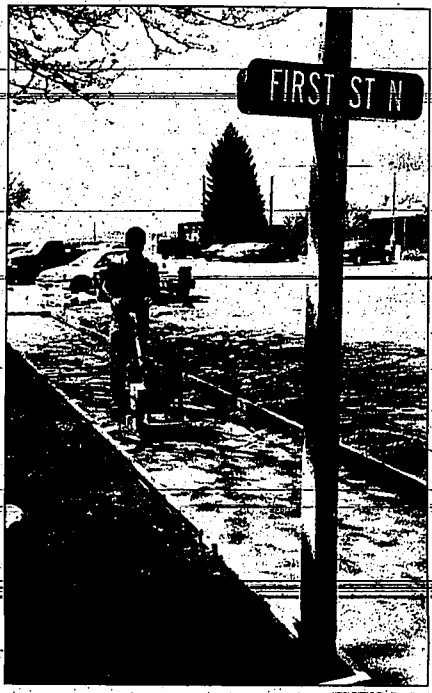
Cree Jones, with Gary D. Jones Construction in Burley, works on a new sidewalk outside the Church of Jesus Christ of Latter-day Saints in Minidoka. The sidewalk will be pulled up so four new straightaways could be installed for safety purposes.
