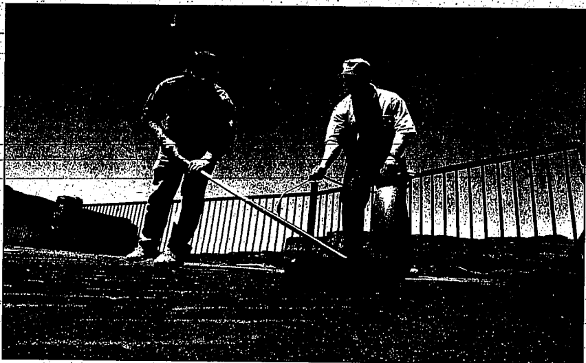
Clint Kiser, right, sprays a wear coating on the new asphalt walkway overlooking the falls at Shoshone Falls Park while Bert Heath spreads the coating with a broom. The two were performing some of the final touches to the park before it opens Saturday.
