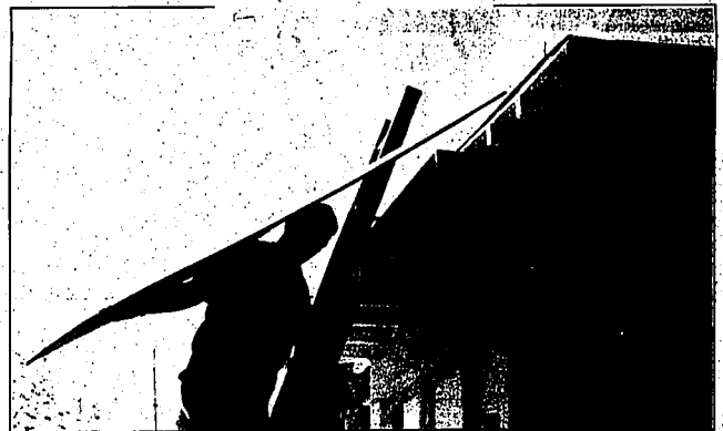
Cody Davis gives a Rupert home a new roof.
