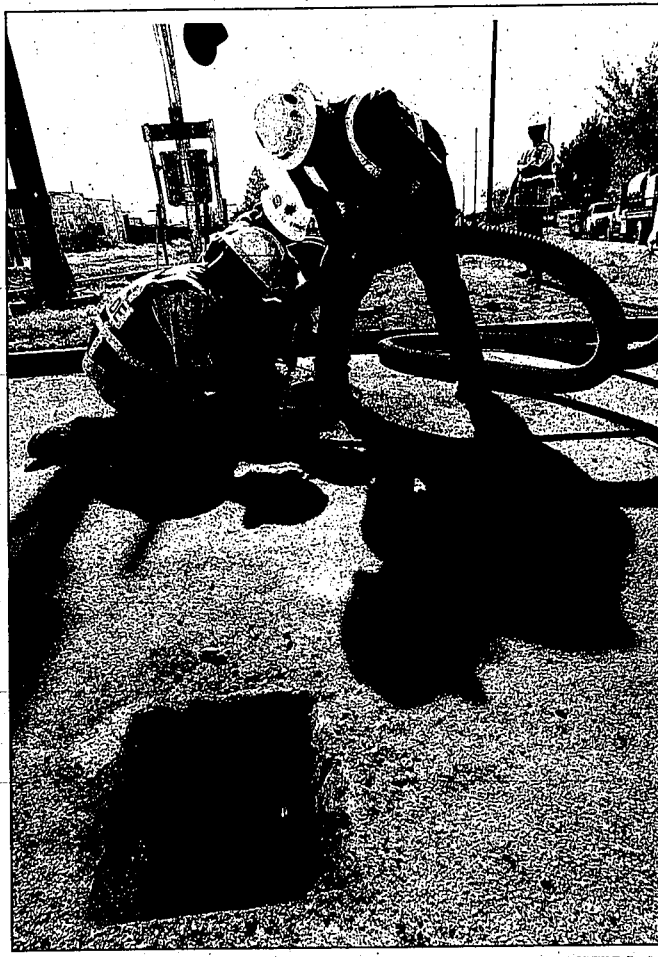
Workers from MaaTec bore a hole into Blue Lakes Boulevard South this week at the intersection of Kimberly Road to prepare for running a fiber-optic cable under the street. Syringa Networks LLC, based in Rupert, plans a 1,419-mile fiber-optic network to link rural southern and eastern Idaho communities with high-speed video, voice and data transmission capabilities - and to attract high-paying jobs. The MaaTec work is part of the Syringa project and, when completed, will include a network from Burley to Bliss.
