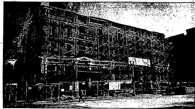
The International Spy Museum, seen Monday and set to open next spring, is going up behind a facade of shops in Washington built in the mid-1800s. The new museum will occupy the first three floors of this building across the street from the National Portrait Gallery and less than a block from the FBI.
