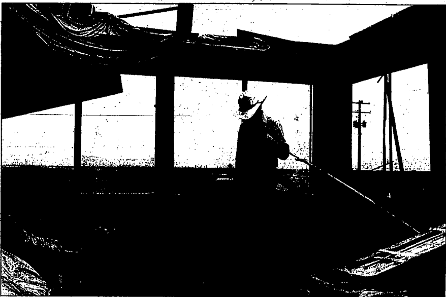
Grant Fehlman, who lives east of Malta, inspects the damage that heavy winds and rain did to his house Thursday. Fehlman, who was waiting for his insurance adjuster to arrive Friday morning, says the house is beyond repair.
