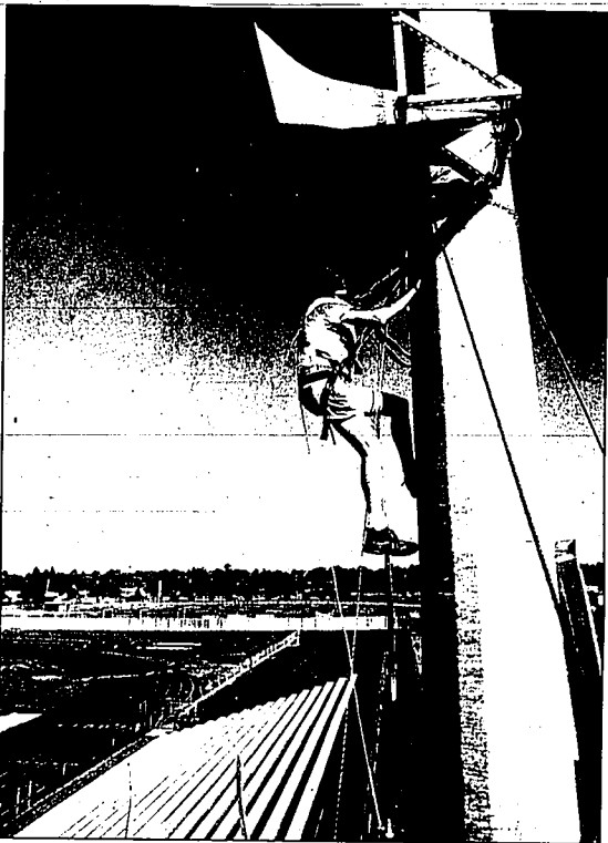
Keith Lee, a worker with Metcalf Electric Inc., attaches a loudspeaker to a light pole at Twin Falls High School. A wooden pole at Bruln Stadium was replaced earlier this year by a metal cell phone tower so the lights and speakers had to be reattached to the new pole.
