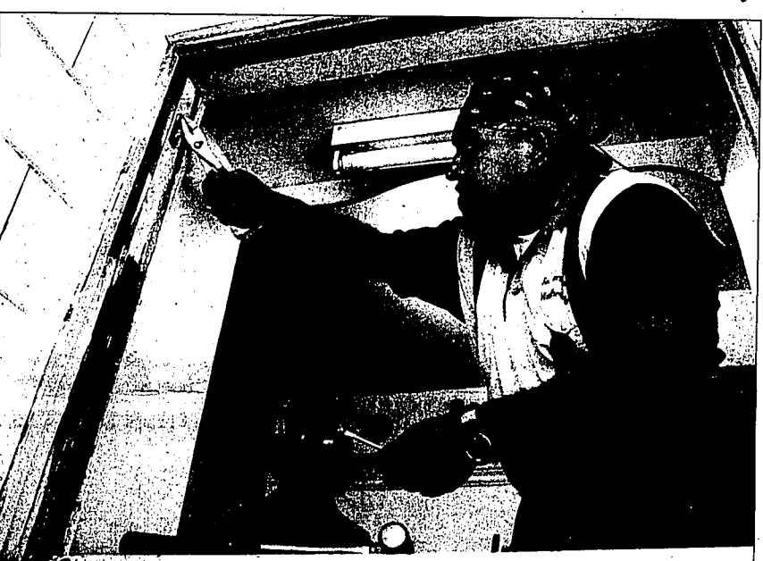
Volunteer Edna Egner watches as Ed Compa replaces a window at the Ike Kistler Safe House administrative offices in Twin Falls on Tuesday afternoon. Compa works for the South Central Community Action Agency, the group responsible for installing about $17,000 worth of weatherizing improvements to the two buildings of the shelter for homeless children.
