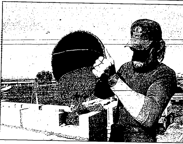
Tony Stauffer works on the new restroom and shower facility under construction at the Heyburn RV Park. Stauffer, mason of Heyburn is doing much of the work at the city-owned facility. Heyburn city officials believe the addition of restrooms to the RV park will increase business, and in turn, revenue to the city.
