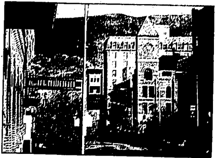
Buildings cast shadows last month in uptown Butte, Mont. A century ago, Evel Knievel's hometown of Butte was "the city that electrified a nation" with wire from its copper mines. Butte was famous for its raucous, bustling streets, sometimes dangerous but always exciting, hard against a mountain of copper ore that was steadily chipped away by miners.
