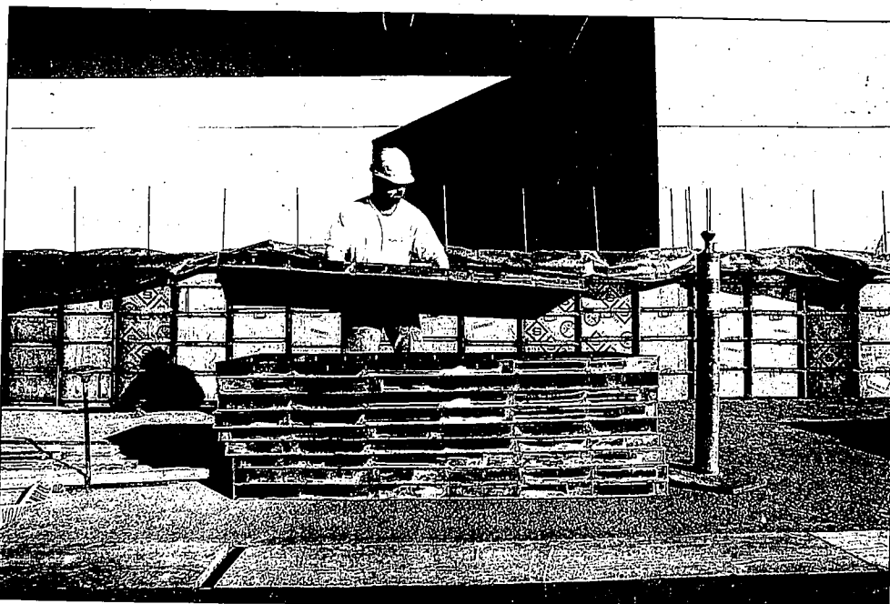
Pat Brown stacks a concrete form taken off a new concrete wall at the WinCo Foods store in Twin Falls. The discount grocery store is adding 5,000 square feet to the existing building and taking over nearby space that other businesses had occupied.
