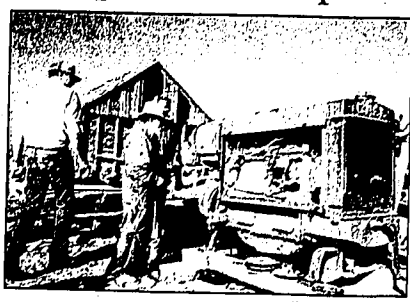
LeRoy Fairchild, center, examines the engine which ran the old sawmill in the Oakley Basin, while volunteers dismantle the mill. Wally Blacker, left, is one of the volunteers as is John Firth, behind Fairchild. The mill was sold to Pioneer Village museum in Utah.
