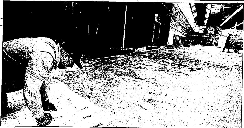
Plumbing contractor Tracy Harr looks over the floor plans for plumbing in the former Polo Line Road Albertson's grocery store, which is being renovated for use by Dell Computer Corp.'s new technical-support operation in Twin Falls.
