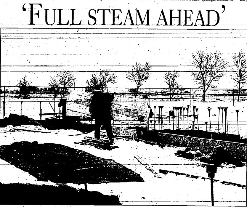
Workers from Kreizenbeck Constructors, Inc., continue to work on the additions at Minico High School. When finished, the school will have a new wing on the front of the building and an additional multi-purpose building.
