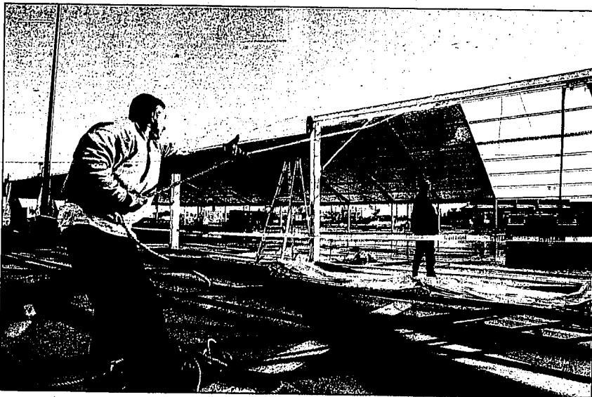
Victor Salazar hauls on a rope that will be attached to a sheet of canvas that goes on the roof of an immense tent being erected in front of the new Dell Computer Corp. call center. The tent will house live entertainment for Saturday's Olympic torch celebration.
