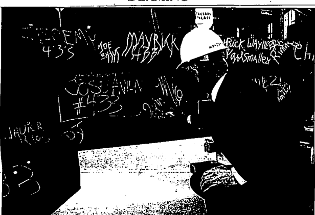
Caesar's Palace President John Groom signs his name to the final beam of the new Colosseum Showroom during a topping out ceremony at Caesar's Palace in Las Vegas Friday. The 100-foot-high showroom built to resemble its Roman namesake is due to open in March 2003.
