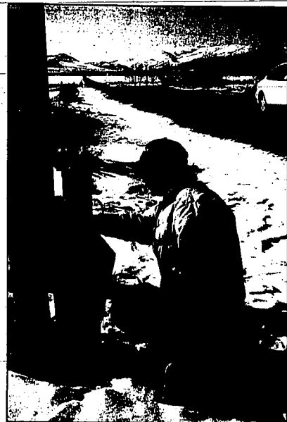
Alblon Telephone Co. technician Darren Smyer checks a noisy residential phone line southeast of Malta Monday afternoon. Melting snow seeping into the lines causes static, he said. Finding the problem area under the snowdrifts could be tricky, Smyer said.
