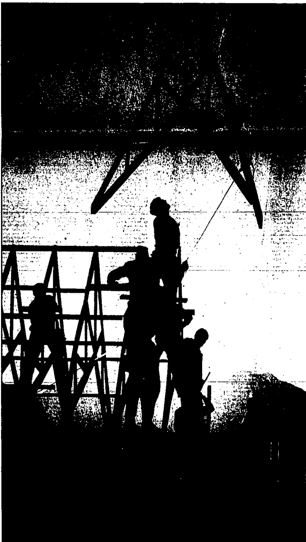
A crew of Mennonites install a truss during construction of the Sangre de Cristo Mennonite Church in Westcliffe, Colo. They came from as far away to 'frolic,' in the language of the church, which means they came to raise a church.
