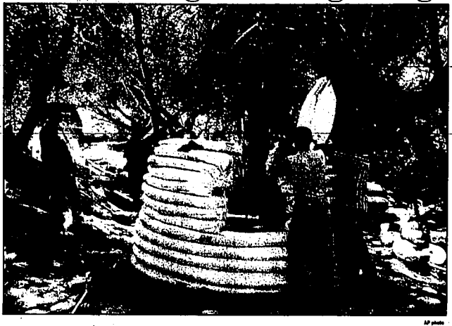
Workers erect a new and temporary housing for migrants, who call it much better than former living conditions.
