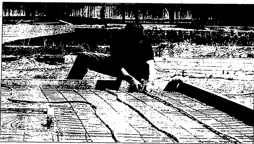
Burley resident Dennis Rose works Thursday afternoon to install pipes, which will heat the floor of his new home. Rose is constructing much of his new house himself. Construction values around Magic Valley are on the rise.
