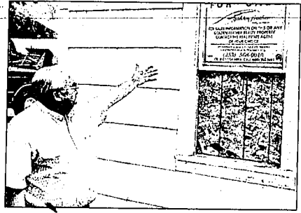
Orville Rotho, president of the Mini-Cassia Shelter for Women and Children, examines windows in the house the city of Rupert may donate to an organization to become a domestic violence shelter. The windows and window frames need to be replaced, he said.
