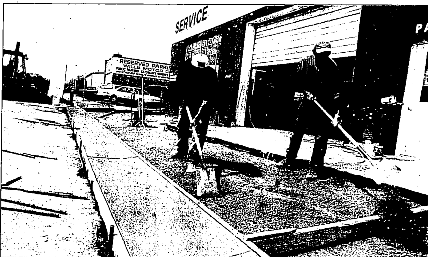
Kelly Thompson, left, and Kip Kytlo work on the new sidewalks at Willis Toyota in Twin Falls Friday. The sidewalks are one of several construction projects on the property, including a new service bay with a lift.
