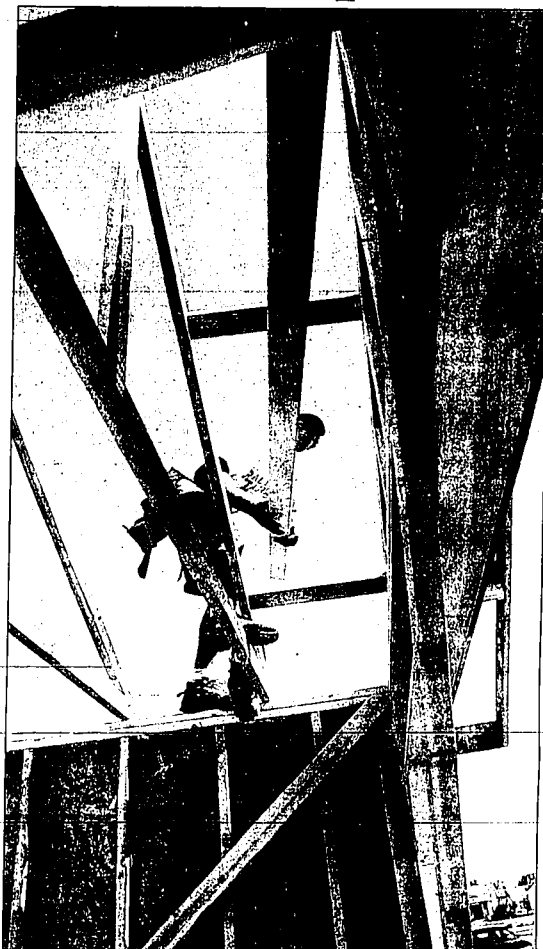
Chris Hoy, owner of C&A Construction, works on securing dry-wall backing on a garage frame for a new single-family home in Twin Falls.
