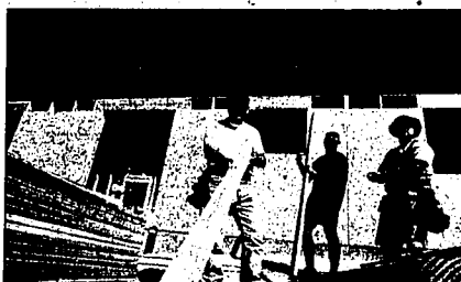
Kent Murphy, left, picks out a straight board for use in his house while Matt Jeske and Tom Daniels, right, help out. All 10 houses had to be ready to occupy before any of the residents could move in, so everyone pitched in on all 10 houses.
