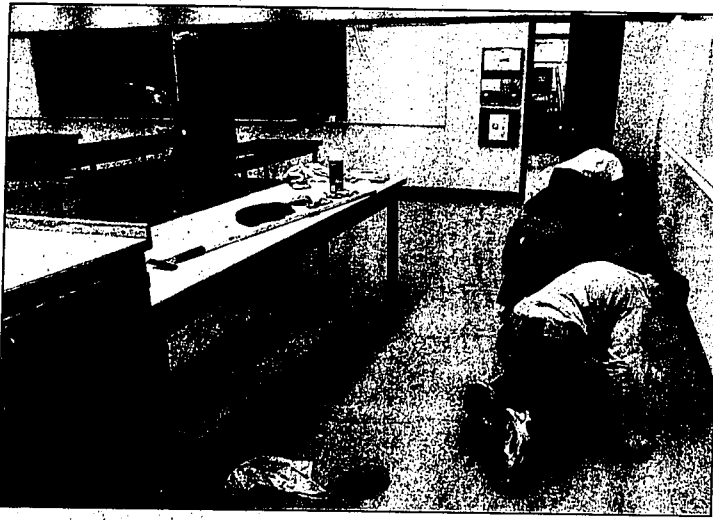
Merlin Blake, left, with the College of Southern Idaho maintenance department, puts some finishing touches on one of the new biology classrooms at CSI while other custodians scrub paint from the floor. Several science classrooms in the Shields Building have been remodeled this summer to accommodate the increased number of students enrolled.
