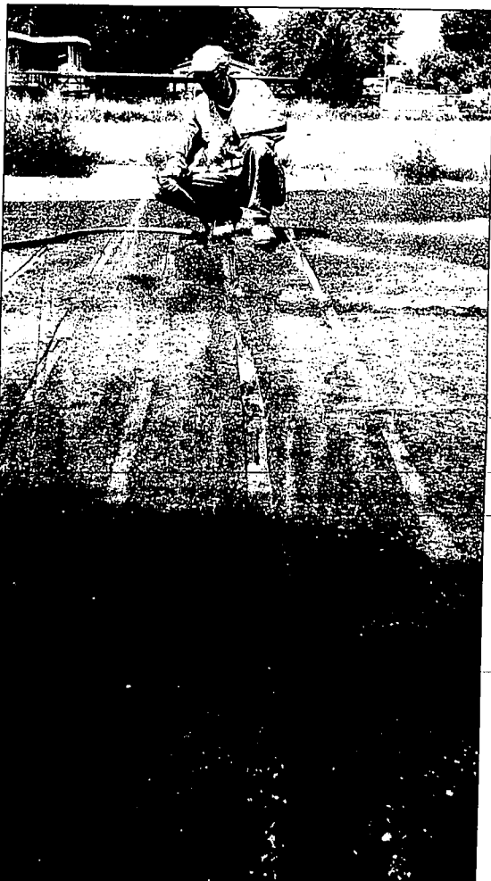
Jeff Bay, a worker with A-Core of Magic Valley, washes debris out of grooves he cut in the pavement on Locust Street North in Twin Falls Tuesday to warn drivers they are entering a school zone. Plans call for 76 more sets of rumble strips on city streets.
