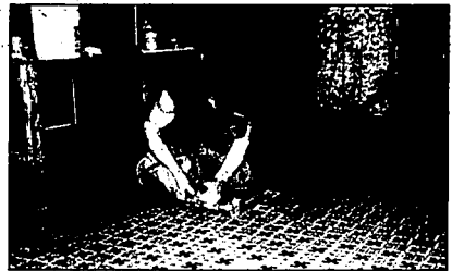
Kevin Heffner works to clean layers of glue off the old tile floor at the Drift Inn in Rupert. Renovation started with a disc jockey "The Vault," which will feature live entertainment, karaoke and disc bucks on Saturdays.
