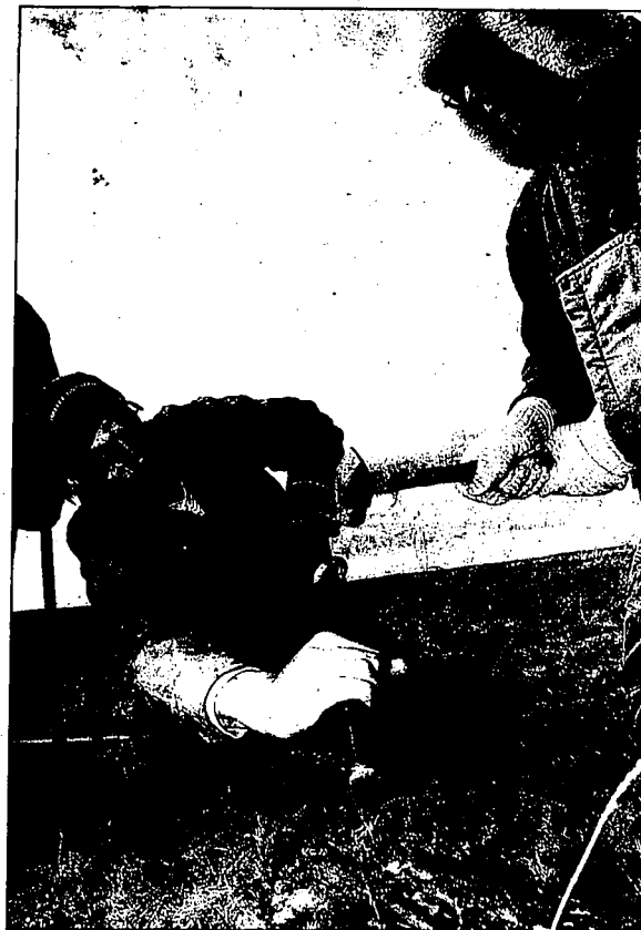
Rommie Jarolimek, a person interested in wind power, and Gerald Fleischman, staff engineer for the Idaho Energy Division, work Monday to secure one of four anchors, where guy-wires were attached, which will hold an anemometer in place. The anemometer, south of Kimberly, will test wind potential.
