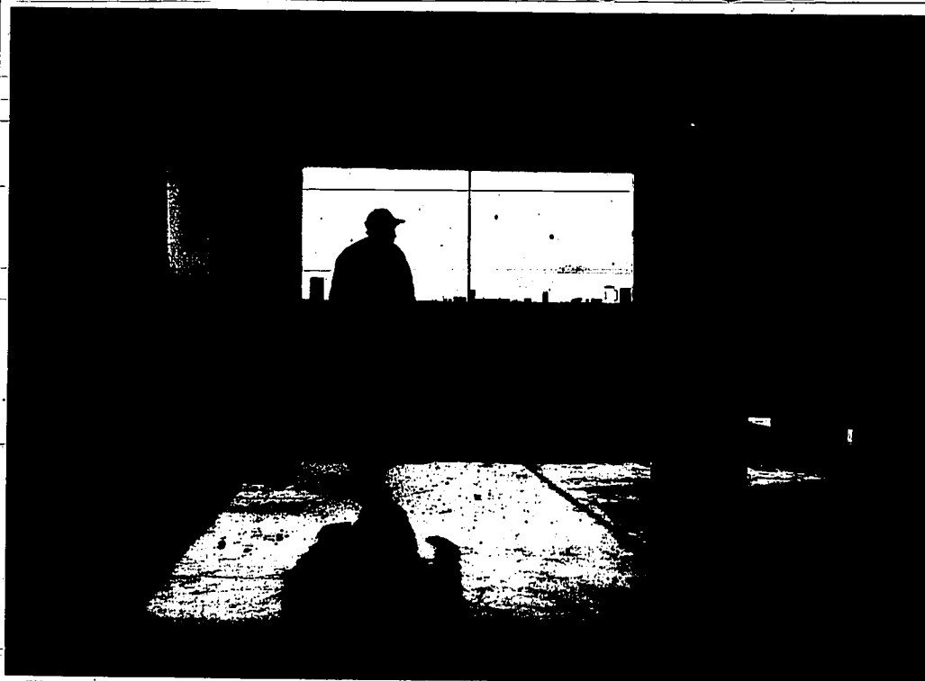
Lane Lucas, a worker with Don Anderson Construction, walks through what will be the lobby area of a professional office building when crews finish renovating the former Gem State Paper warehouse in Old Towne Twin Falls.
